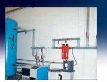
Distribution pipeworks in aluminium for compressed air, vacuum and other non dangerous gases, from 20 to 110 mm diameter.
